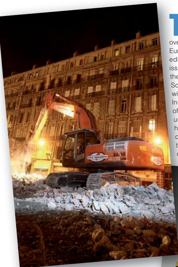
DSD Démolition is currently demolishing the A55 motorway bridge in Marseille. It has three large Hitachi excavators, a ZX450LCH-3, ZX350LC, and ZX350LCN-3, working round the clock to complete the task within three months
